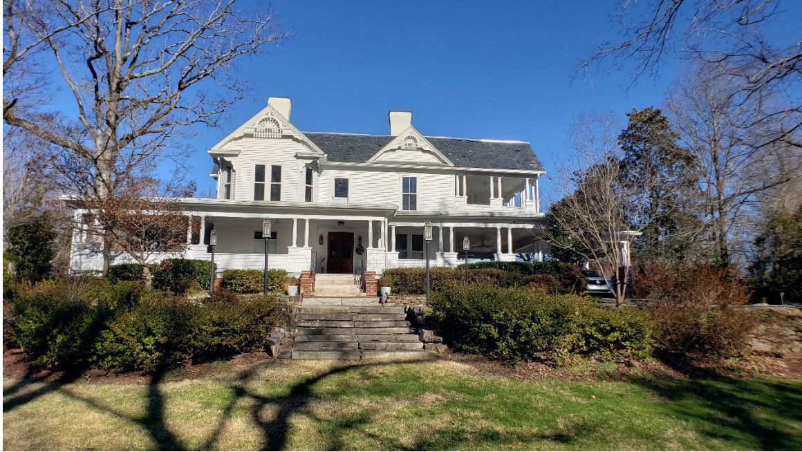
Existing House: View from Union Street South
